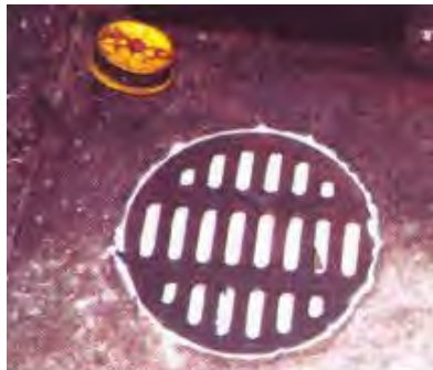
A common source of pollution from businesses is a floor drain that is improperly connected to a storm drain (Source: Petro-Marine Company, Inc., no date)
