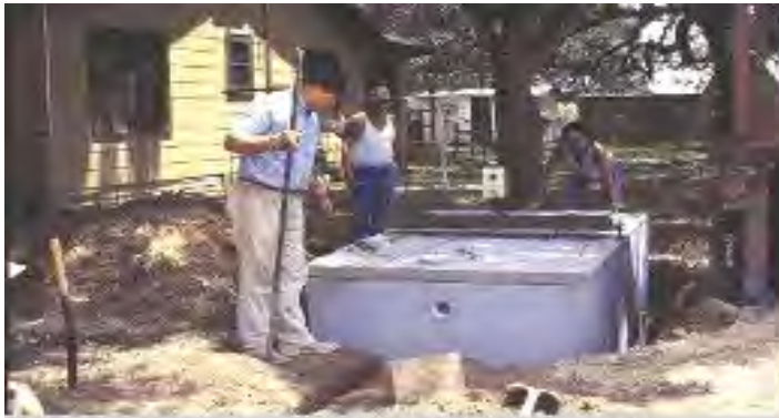
Many times an aged or failing septic system requires tank replacement (Source: Texas A&M University, 1995)
